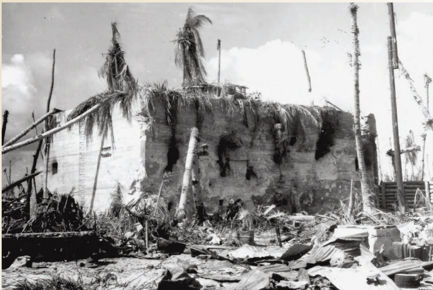
The 3rd Special Konkyochitai command bunker was struck by many naval rounds from 5-inchers up to 14-inchers but none penetrated the structure.
