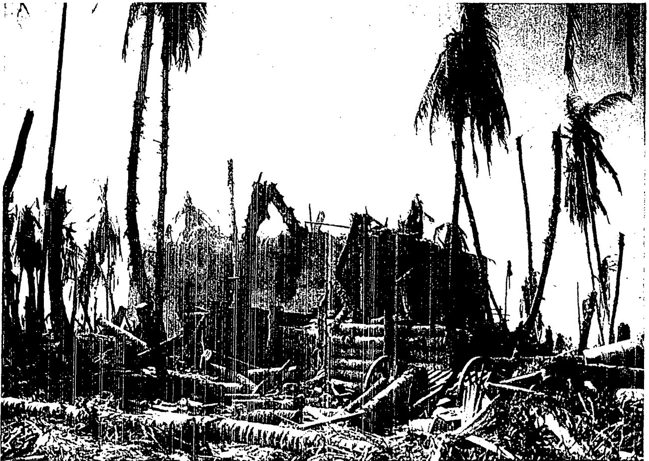
Direct hits from destroyers failed to demolish this blockhouse used as a command post on Tarawa. Constructed of concrete and reinforced with sand and coconut logs, its walls were eight feet thick.
