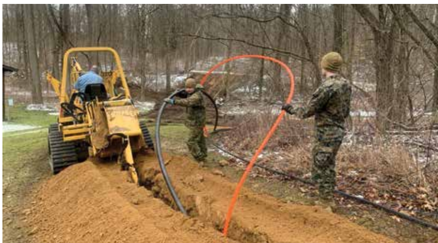
Engineer Services Company, Combat Logistics Battalion 25 Utilities Marines work with John Callan, Scouting American, LaSalle Council to lay conduit. (Photo by GySgt Nicholas Foley.)
