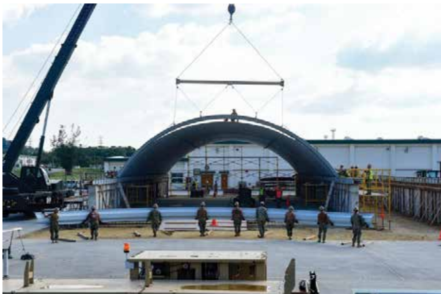
A K-Span is a low-cost and expedient structure that can be built in a variety of sizes due to its modular design. (Photo by Petty Officer 2nd Class Michael Lopez.)
