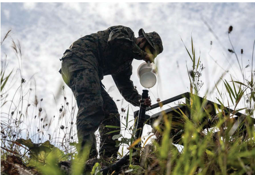
Cpl Taylor, a water support technician with Energy Company, Combat Logistics Regiment 3, primes the raw water pump during Exercise RESOLUTE DRAGON 22 at Kamifurano Maneuver Area, Hokkaido, Japan. (Photo by Cpl Moises Rodriguez.)
