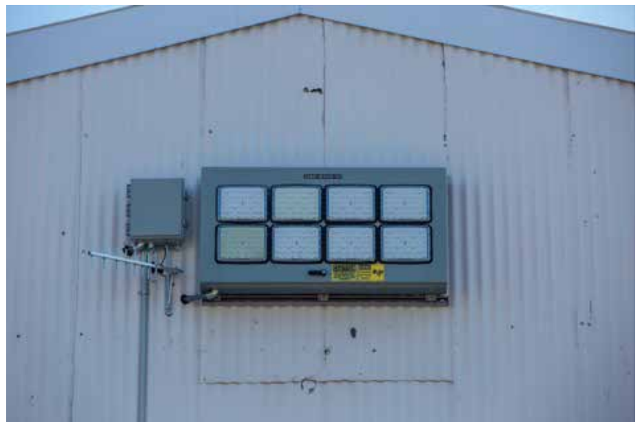
The Lightning Warning Panels provide a visual indication to all personnel on the flightline when lightning is detected within five miles of MCAS New River. This provides realtime warnings for observed hazards to protect the Marines, Sailors, and Airmen supporting the ACE mission of II MEF. (Photo by Cpl Christian Ayers.)
