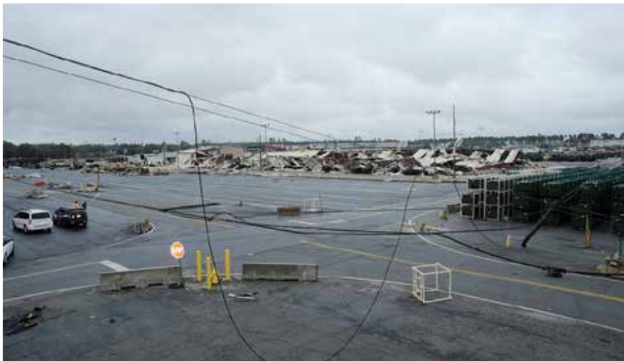
In January 2017, MCLB Albany suffered severe infrastructure damage following a tornado, demonstrating the imperatives for energy security and resilience. (Photo by Nathan Hanks.)
