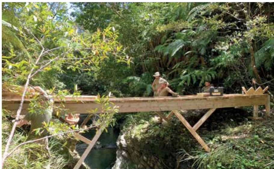
Marine Combat Engineers and Navy Seabees construct a non-standard bridge at Jungle Warfare Training Center, Okinawa, Japan. (Photo provided by B Co, 9th ESB.)
