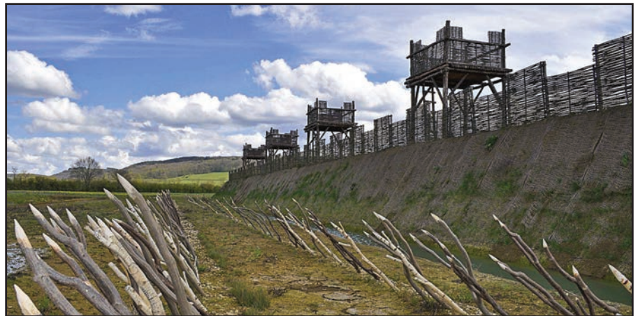
Roman fortifications at Alesia, barrier of stakes with walls and tower behind them.
