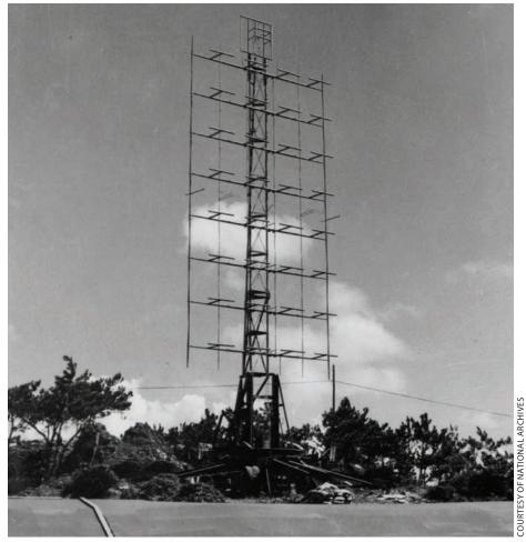
Above: Antiaircraft units on Okinawa used this type of radar array to detect Japanese airplanes during World War II. Hodges, working in the intelligence and operations section, had to quickly assemble and disseminate information from the radar networks and tactical fighter networks to the gun batteries in the unit.
