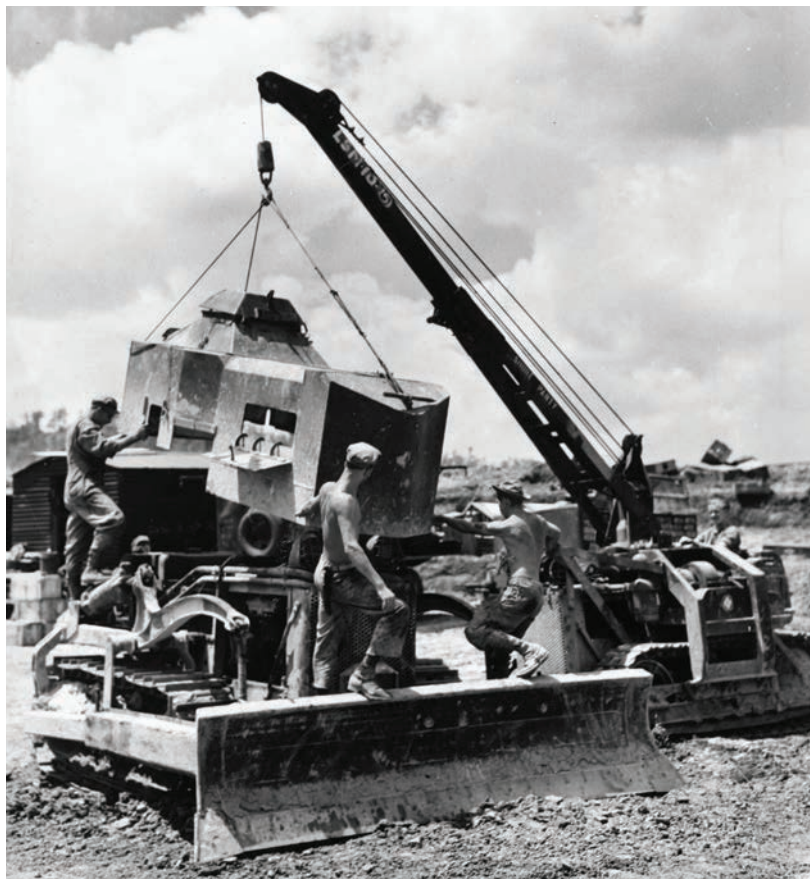
Marines from 1st Engineer Battalion prepare for combat by installing a “suit of armor” on an International TD-9 bulldozer. Drivers were prime targets for enemy snipers, and civilian-built dozers began sporting theater-made armor plating early in the war. While some vehicles were permanently encased, removable kits could be added or removed as needed—an important weight-saving consideration when faced with excessively muddy conditions. (Photo by TSgt Glen A. Fitzgerald, USMC)
