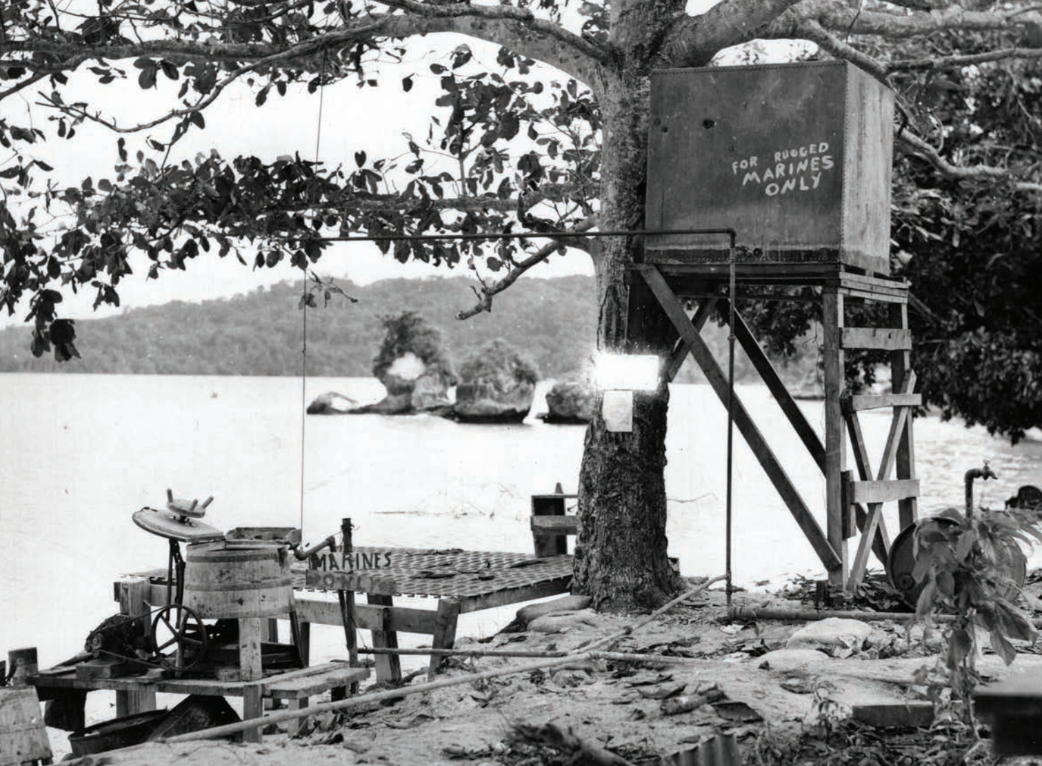
Only "Rugged Marines" were allowed to use this multi-purpose watering station on Tulagi. The main attraction is a shower built from a salvaged tank—complete with a pull chain for easy use. The showering platform appears to be sections of Marston matting. The bucket-shaped objects on the left are washing machines commandeered from Tulagi's Chinatown. At least one is rigged to a motor for automated agitation. (Photo by MG Bert Lynch, USMC)
