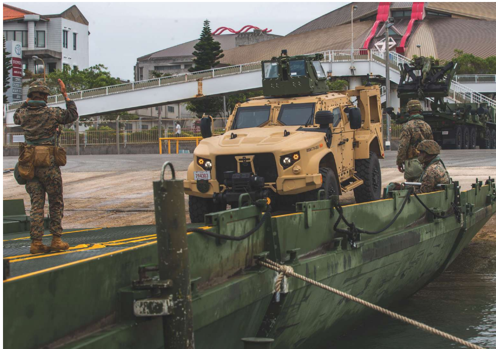
Marines with 9th ESB and Navy Seabees with NMCB-4 load a JLTV onto an improved ribbon bridge during Exercise Pacific Pioneer at Naha Port, Okinawa, Japan, April 21. (Photo by LCpl Alyssa Chuluda, USMC)
