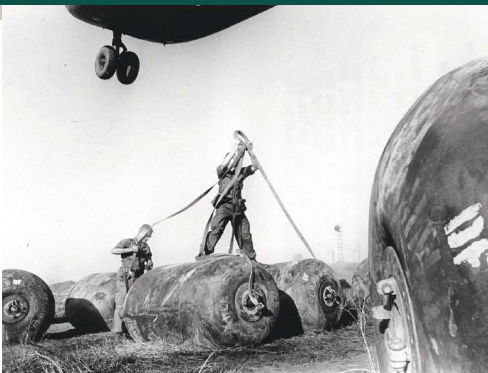
Elephant turd: 500-gallon black rubber (neoprene) fuel bladders carried in 2.5-ton cargo trucks and helicopters, or positioned on airfields and motor pools for refueling. (Photo by Sgt Mike Padillas, USMC)
