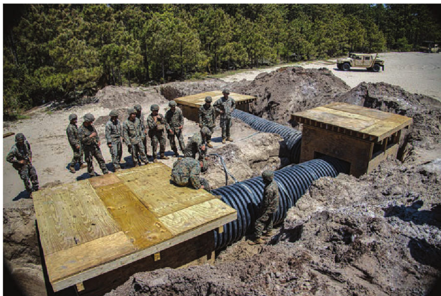
Marines with 8th Engineer Support Battalion complete the construction of underground bunkers during a field exercise. (Photo by LCpl Meshag Hylton.)
