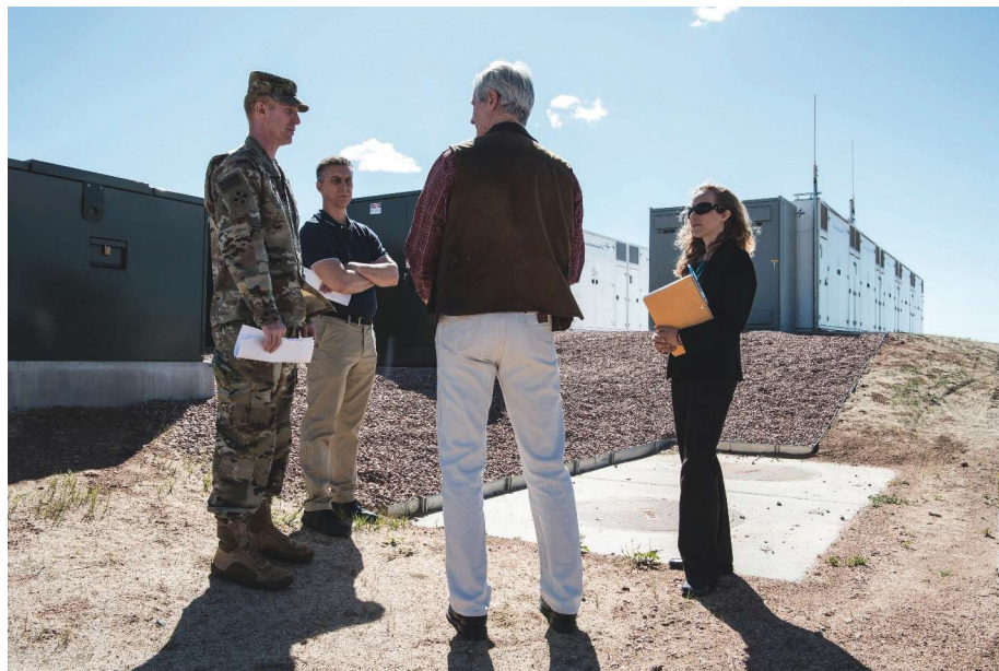
2019—National Renewable Energy Laboratory (NREL) researcher Kate Anderson meets with USA COL Wortlinger, Fort Carson, CO garrison commander, at the base's utility scale lithium ion Battery Energy Storage System (BESS) installation. NREL provided an independent review of Fort Carson's proposed BESS through funding from the U.S. Department of Energy's Federal Energy Management Program. NREL verified the batteries' potential economic savings and helped Fort Carson characterize technology risk. (Photo by Dennis Schroeder/NREL—www.nrel.gov)
