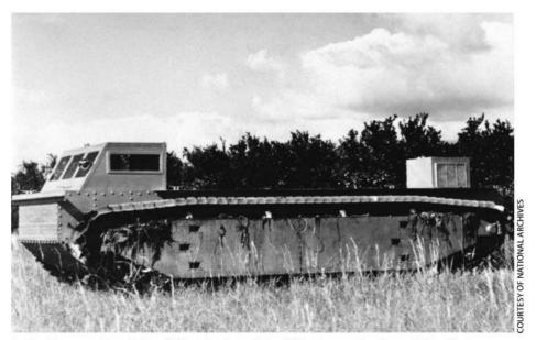
A Florida man, Donald Roebling designed the Alligator so that it could easily traverse the swampy Everglades, and manage to climb back onto shore. Above is one of Roebling's early 1936 versions, while below, a 1937 prototype is being tested.
