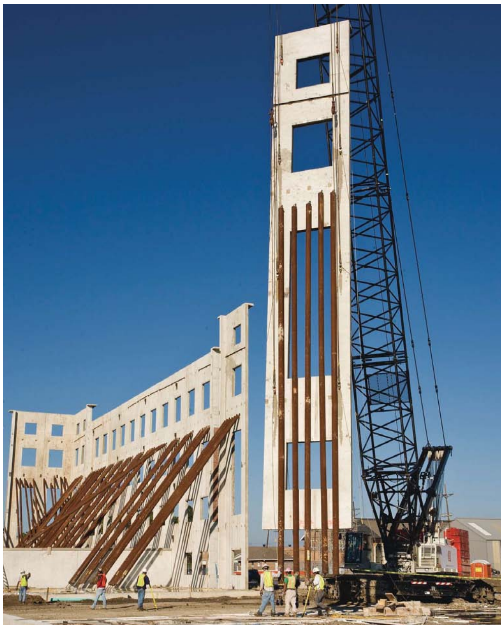
Above: The use of tilt-up construction not only saved millions of dollars, but shaved time off the project schedule. (Jeff Johnston Photography provided courtesy of Woodward Design & Build)
