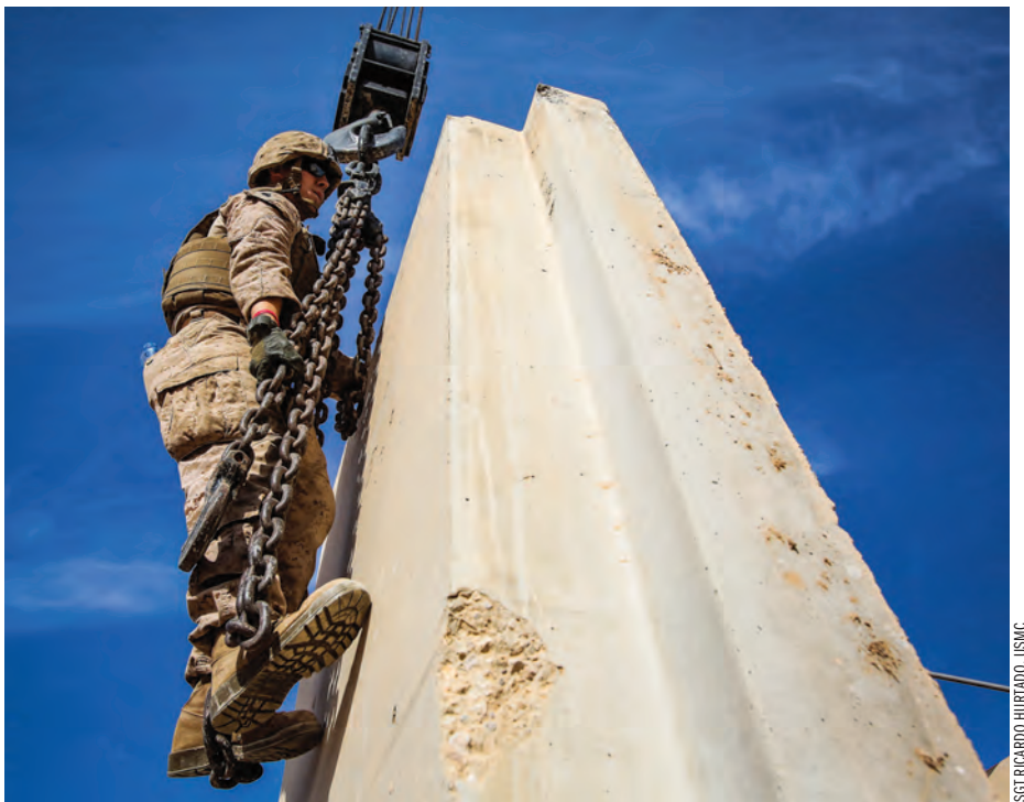
Sgt Edward Hooper, an electrician with Engineer Co, CLB-1, currently deployed with SPMAGTF-CR-CC, attaches chains from the hook block of a MAC-50 crane onto a T-WALL at Al Taqaddum Air Base, Iraq, Oct. 25, 2015. The 12,000-lb. barriers are placed around key structures to provide protection from shrapnel.
