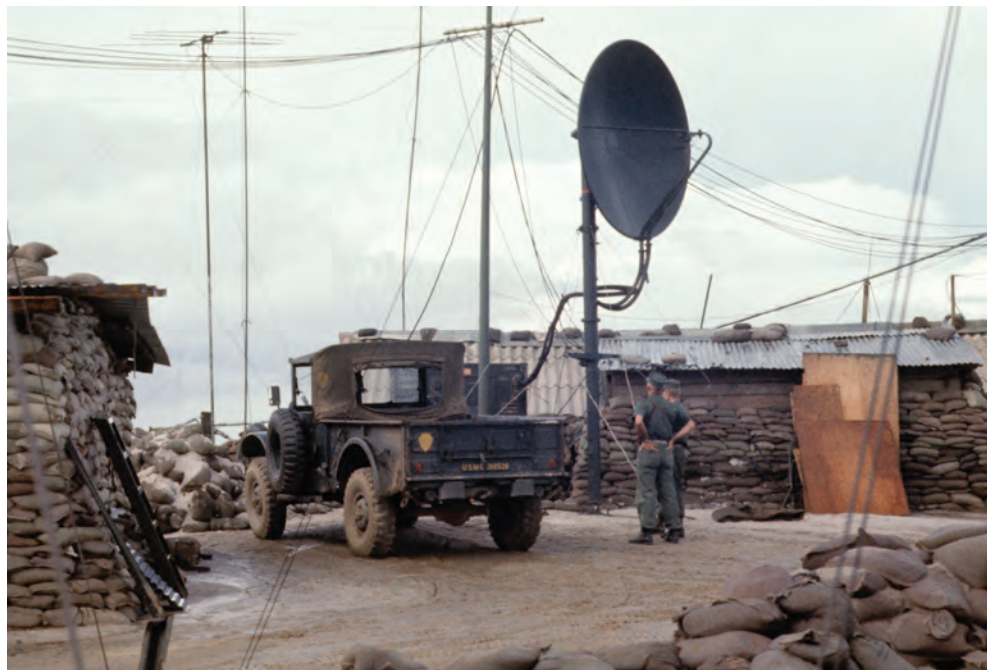
The AN/TRC-97 ("Track 97") long-range radio system, shown here at the Hill 444 Radio Relay Site west of Da Nang, Vietnam, in 1967, was often deadlined. Sgt Webb was instrumental in identifying the issue and ensuring the problem was rectified.
