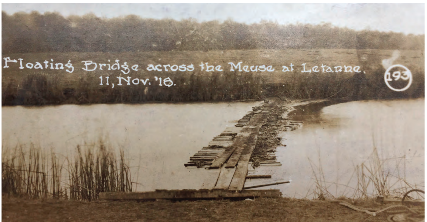
One of two bridges used to cross the Meuse River on the night of Nov. 10, 1918. Note the rough section and the narrow planks for the Marines to walk across.
