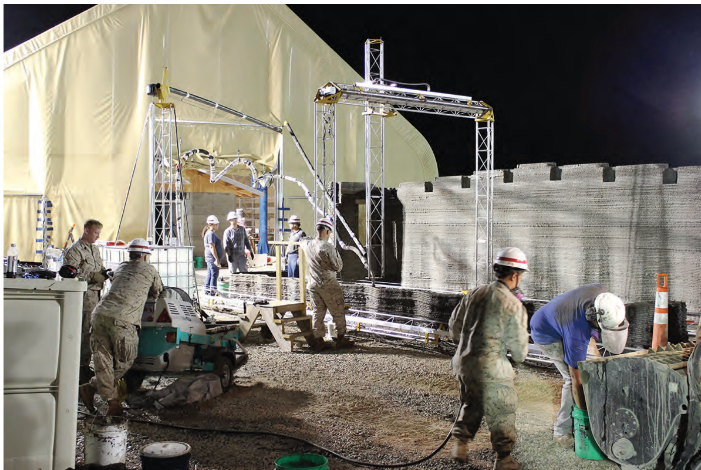
Marines with I MEF learn how to operate the world's largest 3D printer as it constructs a 500-square-foot barracks hut at the U.S. Army Engineer Research and Development Center in Champaign, Ill., Aug. 23. MCSC conducted the field user evaluation to inform future requirements for cutting-edge technology and autonomous systems.
