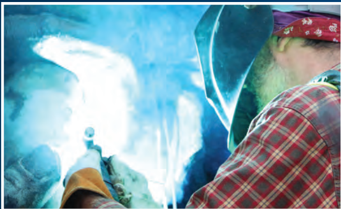
A contractor brazes a portion of the U.S. Marine Corps War Memorial during renovations that took place in the fall of 2017.
