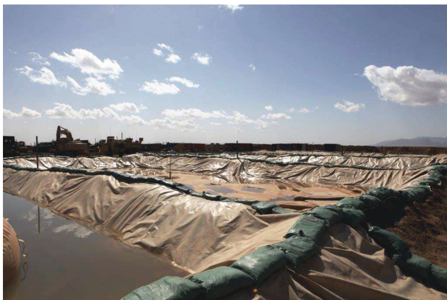
Inflatable storage containers will store fuel to support ground and air operations. (Photo by SSgt John Jackson.)
