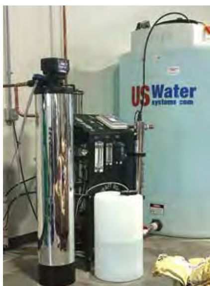
Full Distance Brewing uses a Reverse Osmosis Water Purification system, which removes unwanted chemicals from the water during the brewing process.
