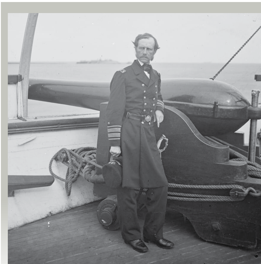
John Dahlgren, pictured here in front of a Dahlgren gun. The gun's large breech drastically tapered down into the muzzle to withstand larger explosive pressures. The guns were nicknamed soda bottles because of their distinctive shape. (Photo courtesy of Library of Congress)
