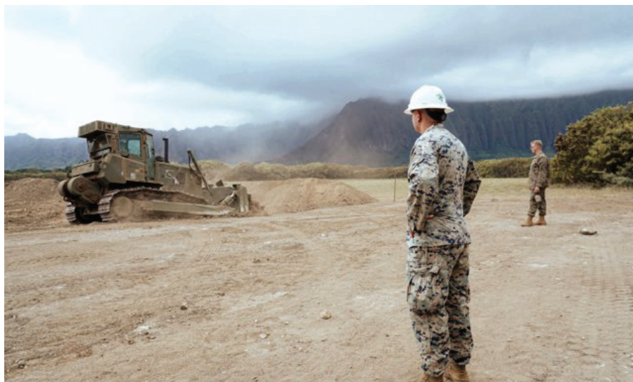
Engineers from an LST conduct earthmoving operations while preparing a forward resupply point. (Photo provided by author.)
