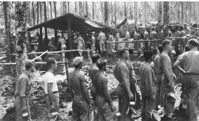
Chow call on Pavuvu in May 1944 for the leather-necks of 1stMarDiv—Pavuvu, the site selected for the Division's rest and refit. The photographer wrote, "This picture was taken before coral and sand had been used to fill in the mud holes."
