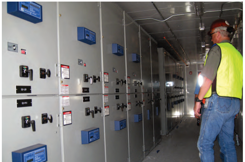
APS reviews the controls in the MCAS Yuma microgrid which eliminates energy interruptions to allow Marines to focus on their aviation mission. (Photo by author.)
